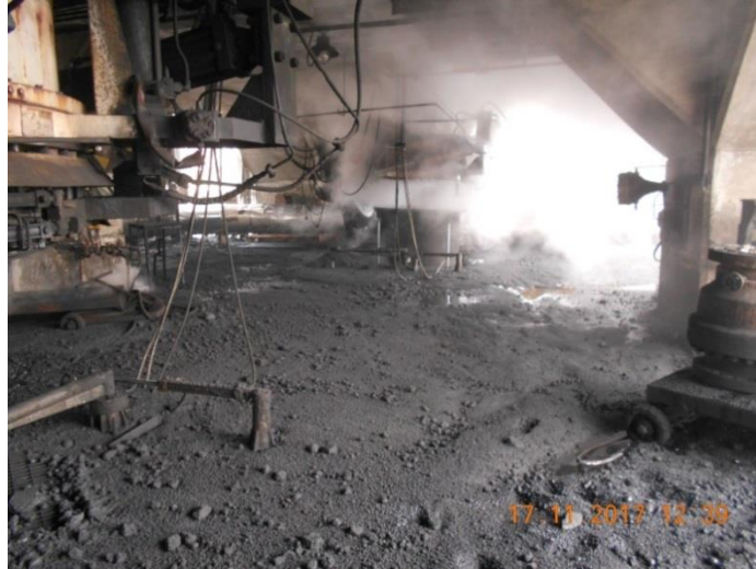
Shot Coke and water spilled on the Switch Deck Platform
