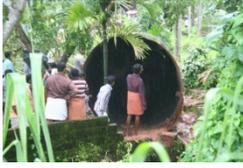
source of ignition is yet to be established. Thereafter, 3 explosions took place consecutively. BLEVE conditions existed and BLEVE probably took place. The front dish end of the bullet with 1/3<sup>rd</sup> of the cylindrical shell of the bullet flew away
